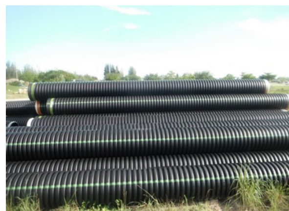
Stormwater Pipes (Black Color Pipes)
