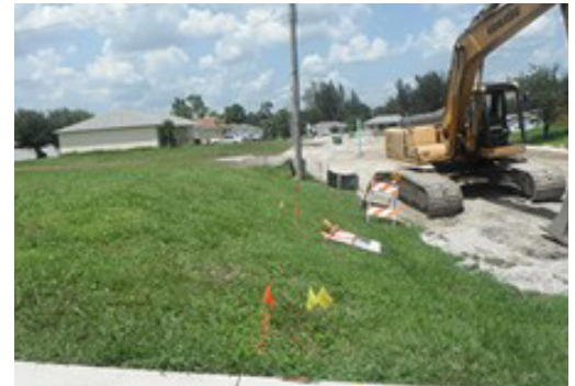
Flagged Utilities in ROW
