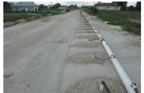
Dewatering Pipes
